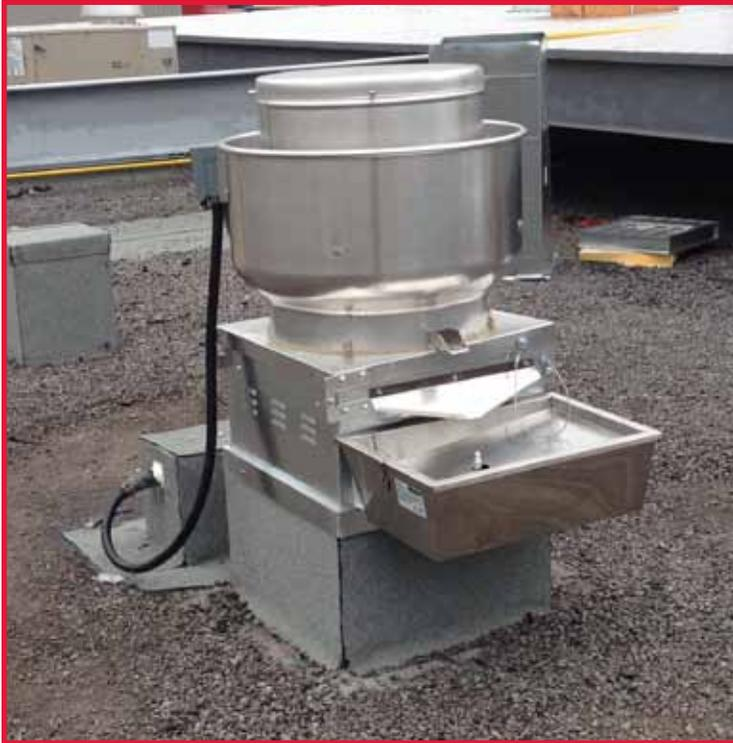
Model EFI-UB shown installed on fan
